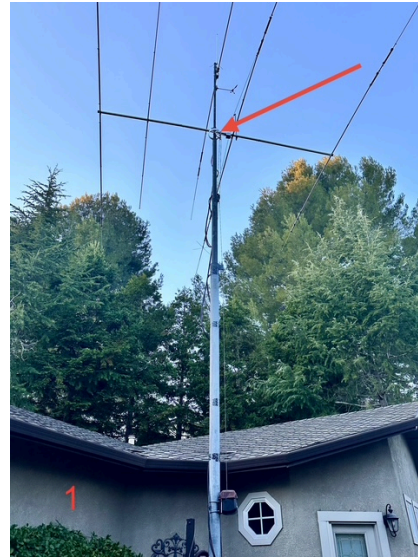
Tower with hand made adapter for 80 m dipole
